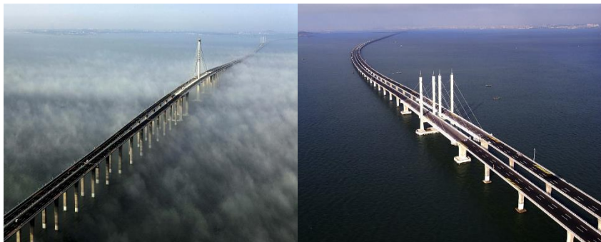
Fig. 4 Podul Danyang Kunshan Grand Bridge
